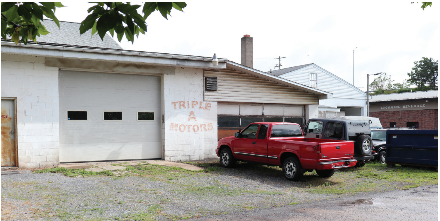
Sherwood Feist moved his free building, one half at a time, to this location.
