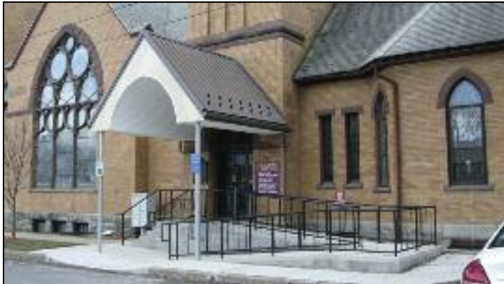
The new canopy entrance at the WECCC.
