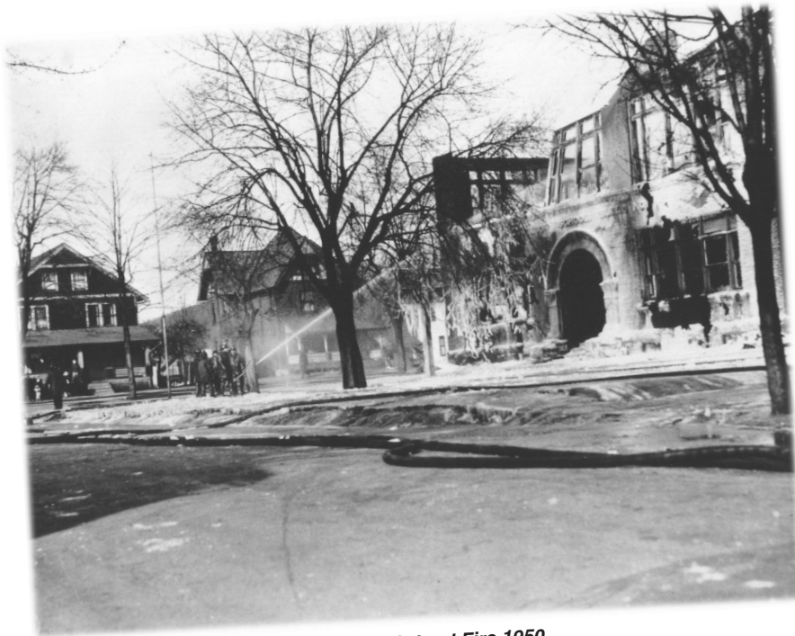
Jackson School Fire 1950 Photo Courtesy of John McDermott
